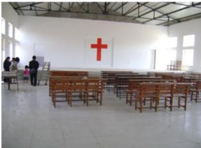
Wangshi Church unfinished sanctuary
